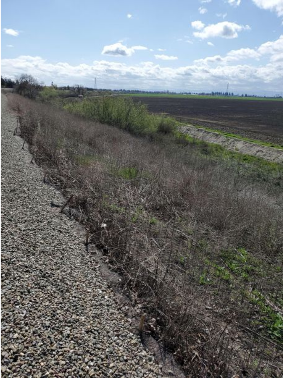
Standing on the levee slope, facing south west.
