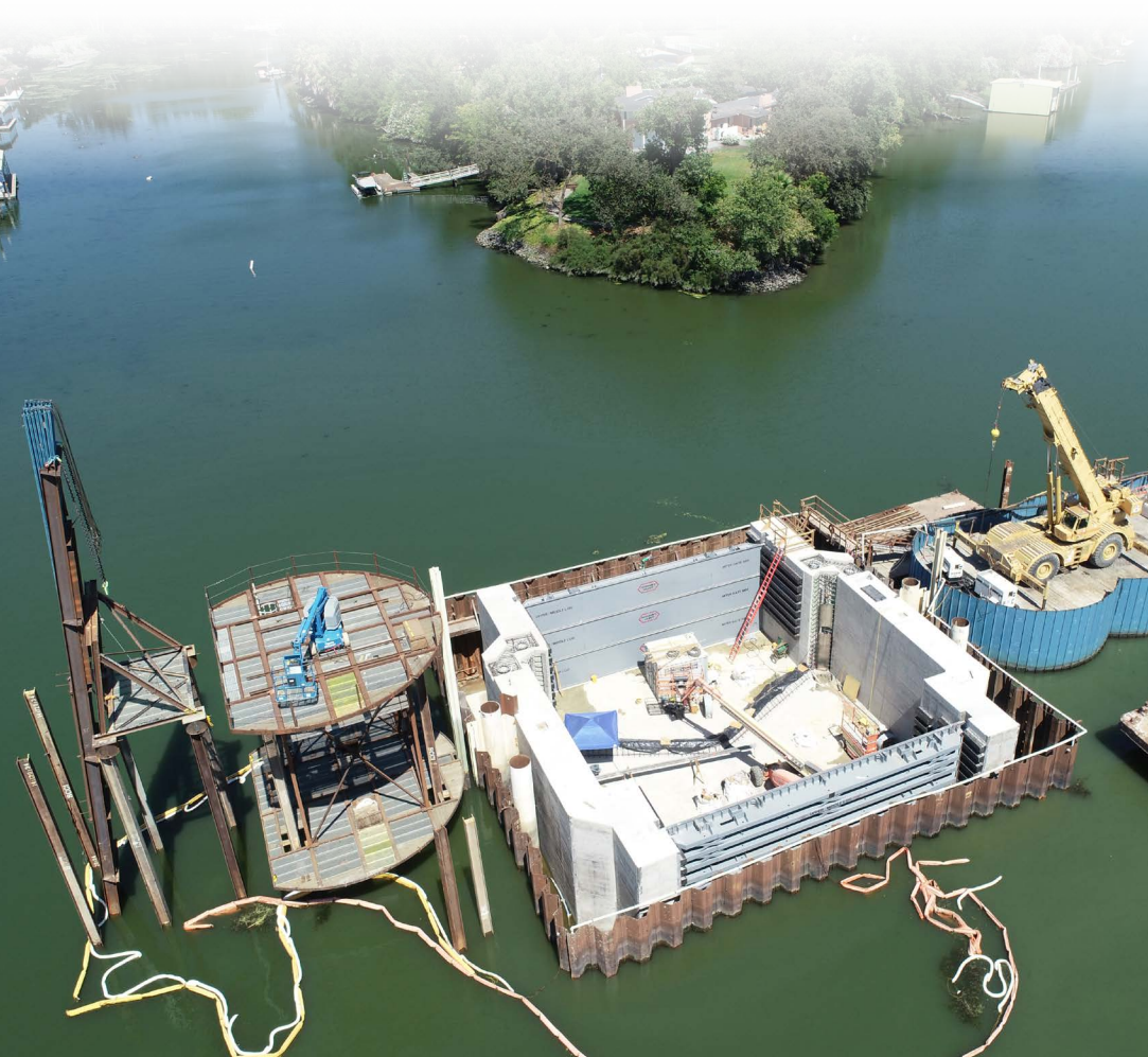
Smith Canal Gate Project - July 2022
